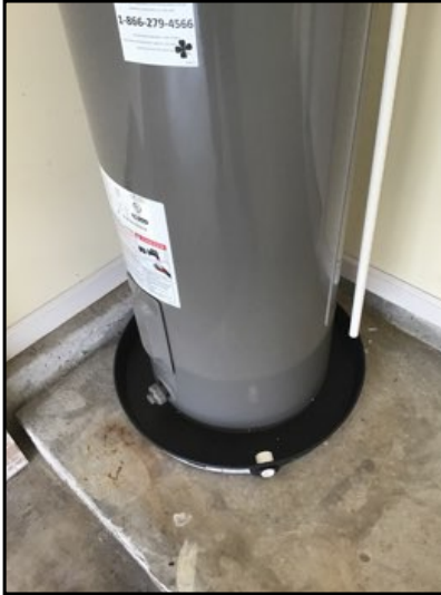
The water heater base is functional.
