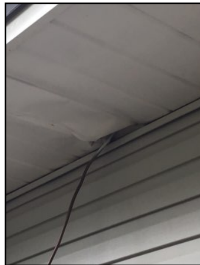
Damaged soffit(s) noted, recommend replacing as necessary.
