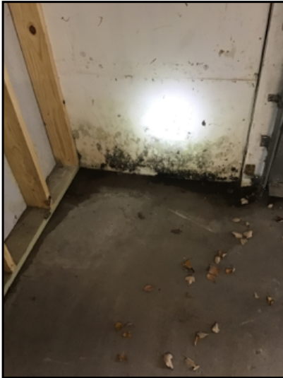
Mold-like bio growth observed. Professional testing & evaluation advised.
