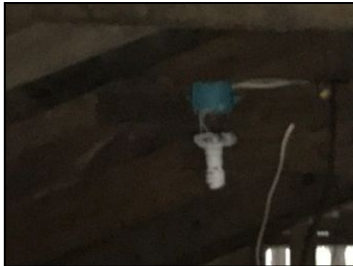
Loose hanging light fixture observed, suggest repairing for safety.
