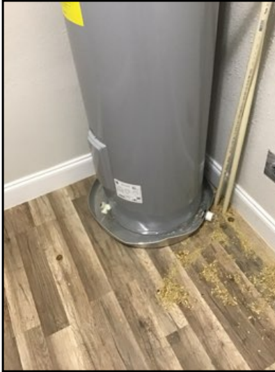
The water heater base is functional.
