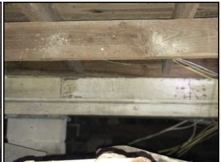
Dimensional lumber wood Joists
