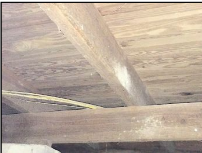
Dimensional lumber wood Joists
