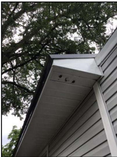
Consider caulking or, at the very least, monitoring for the presence of insects, bird damage, or other activity
