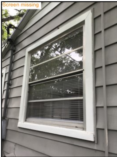
Some window screens missing. Check with seller to determine if they are on the property.
