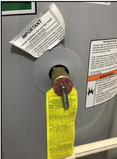
Appears to be in satisfactory condition -- no concerns.
