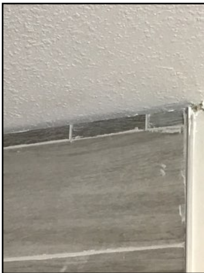
Tile does not extend to the ceiling as gaps are left at the top to collect moisture, recommend correction.
