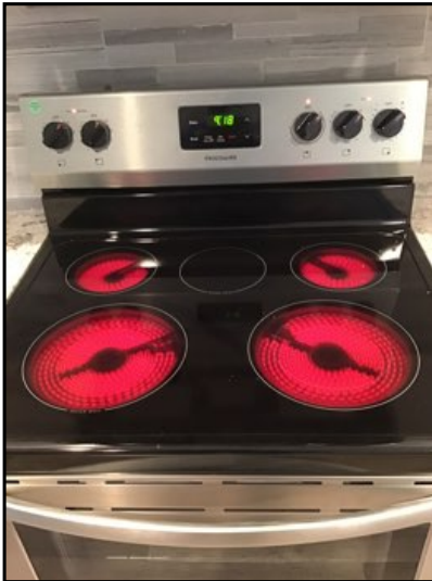
All heating elements operated when tested.
