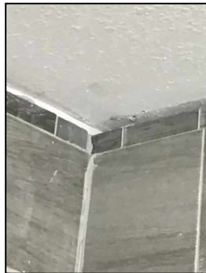
Tile does not extend to the ceiling as gaps are left at the top to collect moisture, recommend correction.
